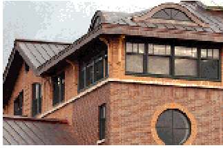
Johnson Hall First Year Residence Hall
